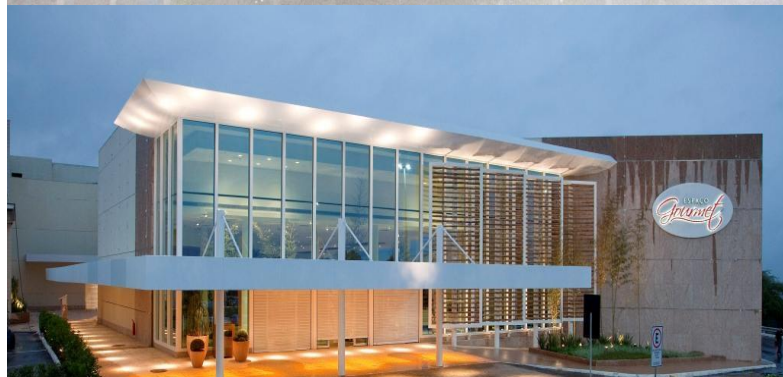
Gourmet Area external view
