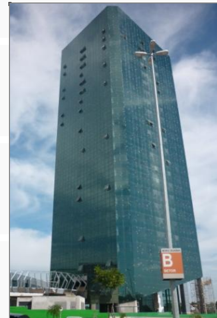
Cristal Tower (RS) Construction site 1Q11
